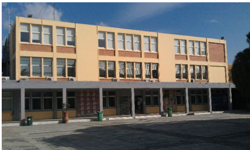
Fig. 6 The case study building
